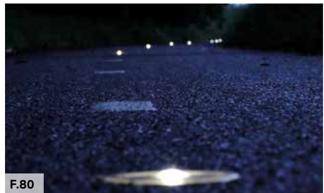
Figure 80: Example of a foot/cycle path which is lit by solar cat's-eye providing some light for pedestrian and cyclists without creating any disturbance to the nearby properties or unacceptable levels of light pollution.
